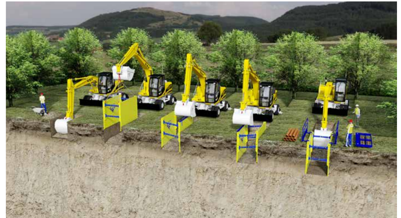
Fig 28: Cut and lower method, using the Standard Box series 600 as an example
