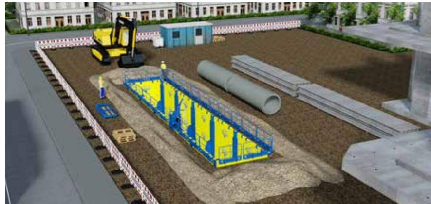
Fig 19: Cut and lower method (depth according to shoring system), no flowing soils
