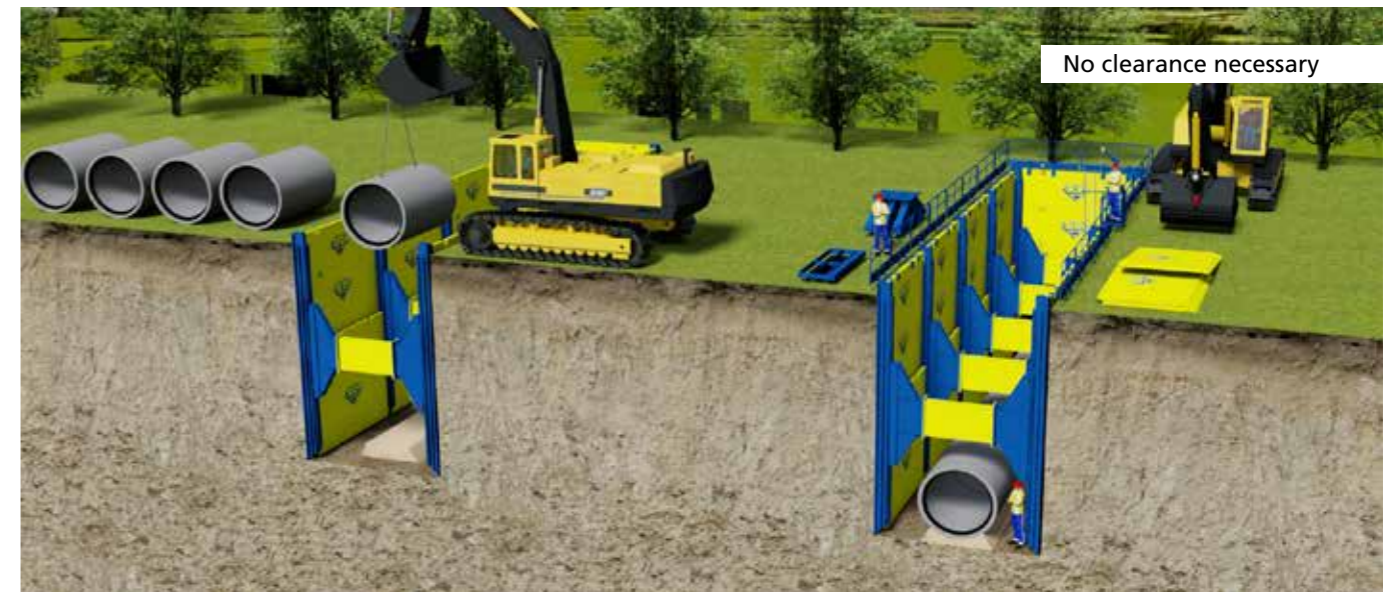
Fig 22: Shored trenches and excavations
