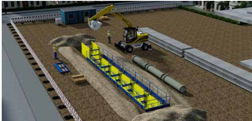
Fig 18: Place and adjust method (depth according to shoring system), for stable or temporarily stable soils
